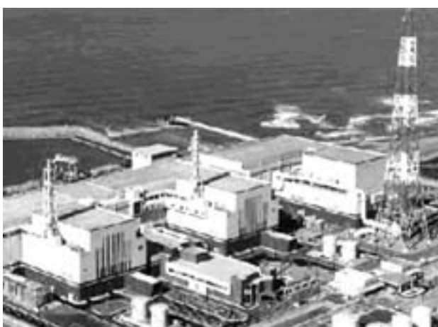
Figura 5. Central nuclear de Kashiwazaki-Kariwa
