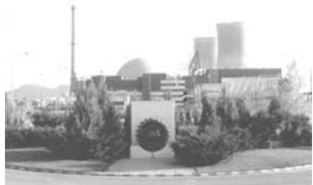
Figura 7. Central Nuclear de Trillo
